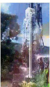
This is the drill rig and crew cleaning out the mud from the drilled well and getting it ready to install the pump. It is always exciting to see the water gushing up from the well!
